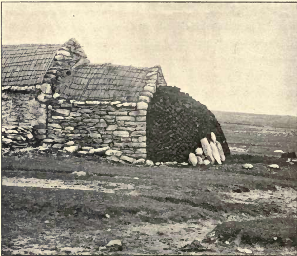
Turf Stack with large stones to prevent wind blowing the turf away, Dooagh, Achill.
